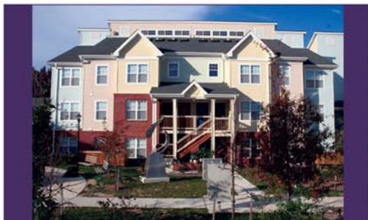
Savannah Heights - This courtyard creates a secure quiet place within a high density inner city multi-family housing development. Sculpture helps to create a sense of place and unique identity.
